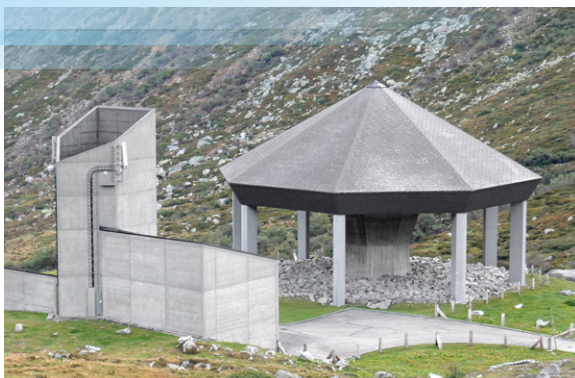
The ventilation stack sits 526 meters above fan no. 21 on the Gotthard Pass.
